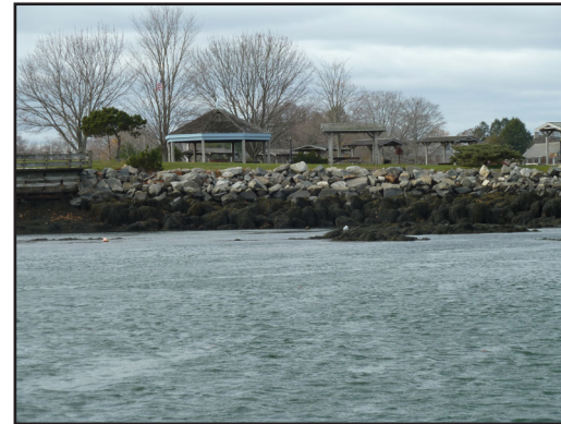
22. Four Tree Island Rip rap at north end of island.
