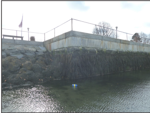
13. At T-Head pier Repoint existing blocks. Water very shallow here.
